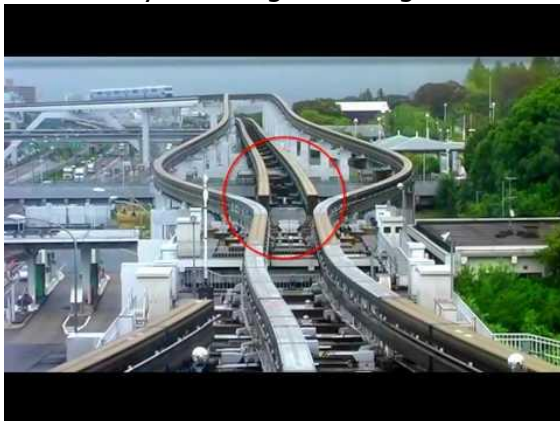
Track Changing Mechanism | Japanese Railroads | Osaka Monorail | JR pass
